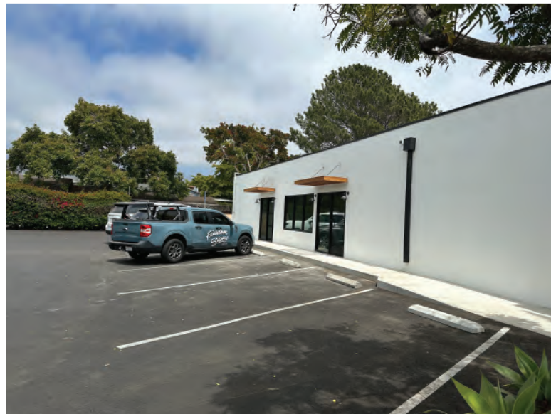
View of units 5032 and 5034
