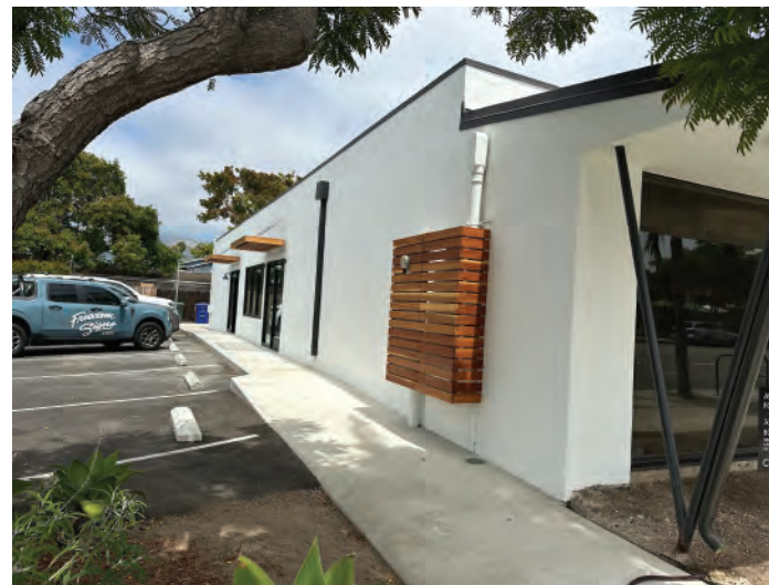
View of parking lot elevation from corner of Carpinteria Ave
