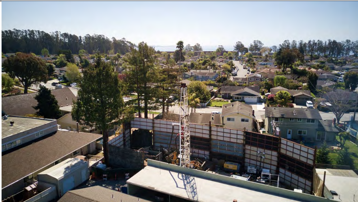
Example Well Drilling Rig with Sound Wall
