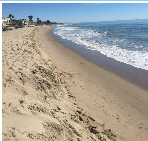
The City installs a seasonal sand berm along the shoreline during the winter season to protect near-shore residences, infrastructure, and Carpinteria City Beach from coastal winter storms.
