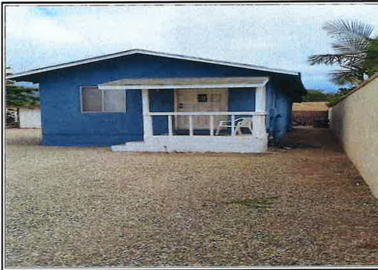
REAR OF SUBJECT PROPERTY
