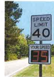
Install dynamic/variable speed warning sign
