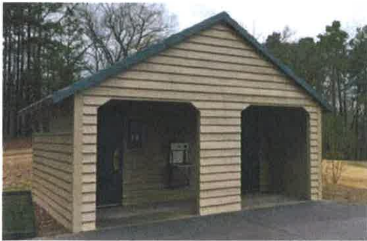
Flush restroom with custom golf cart shelter
