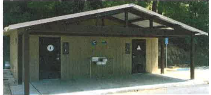
Flush restroom with custom awning
