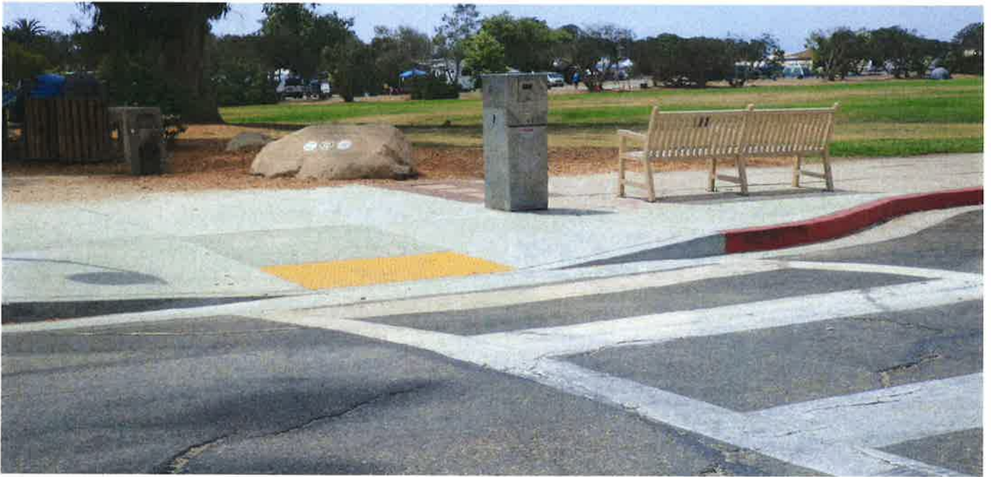
COMPLETED CURB RAMP. NORTH EAST CORNER LINDEN AVE. AND DORRANCE WAY INTERSECTION.
