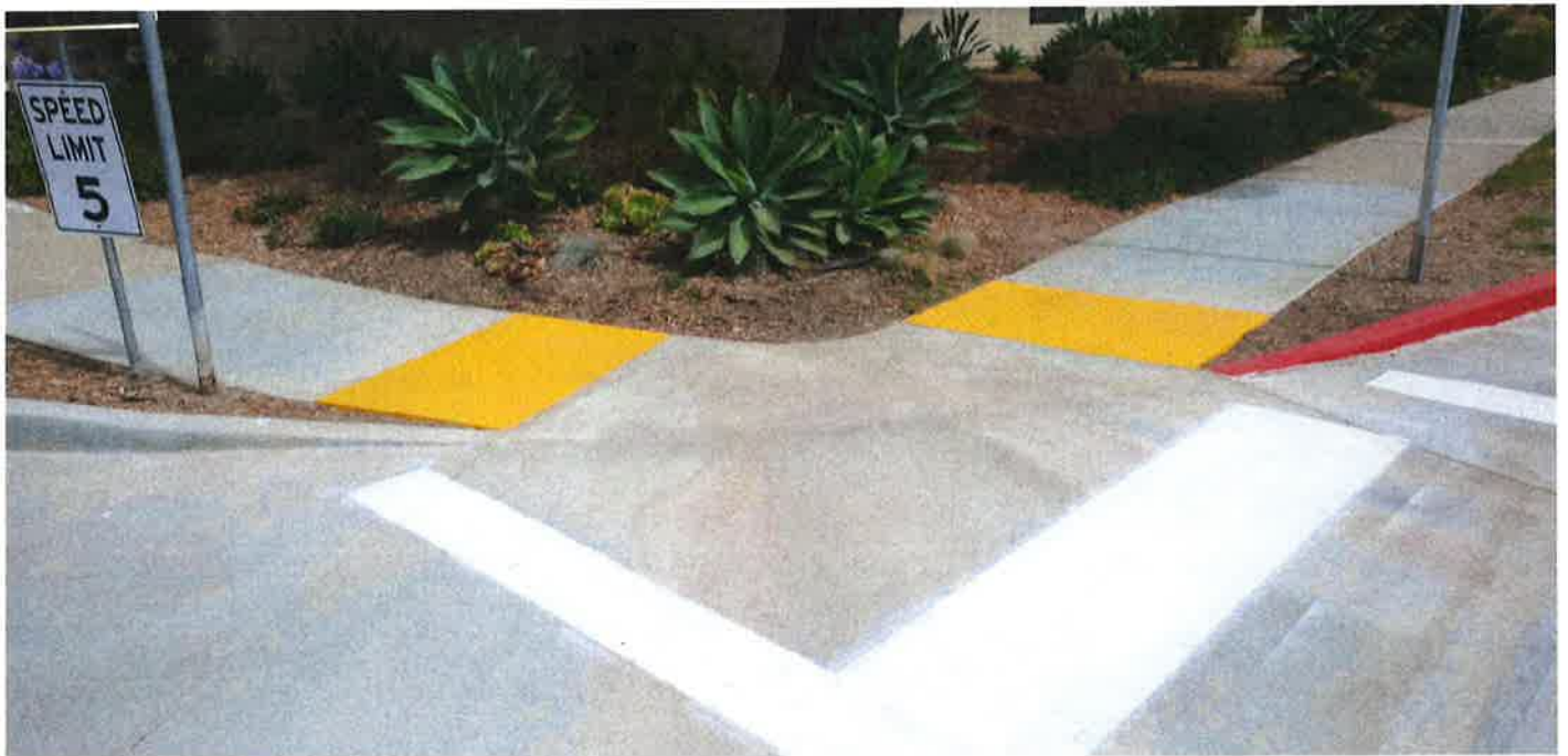
COMPLETED CURB RAMPS. NORTH WEST CORNER SANTA YNEZ AVE. AND CATLIN CIR. INTERSECTION.
