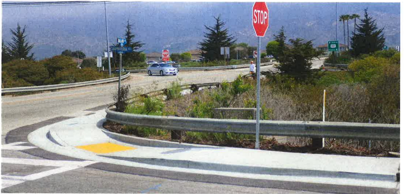
COMPLETED CURB RAMP. NORTH EAST CORNER BAILARD AVE. AND CARPINTERIA AVE. INTERSECTION.
