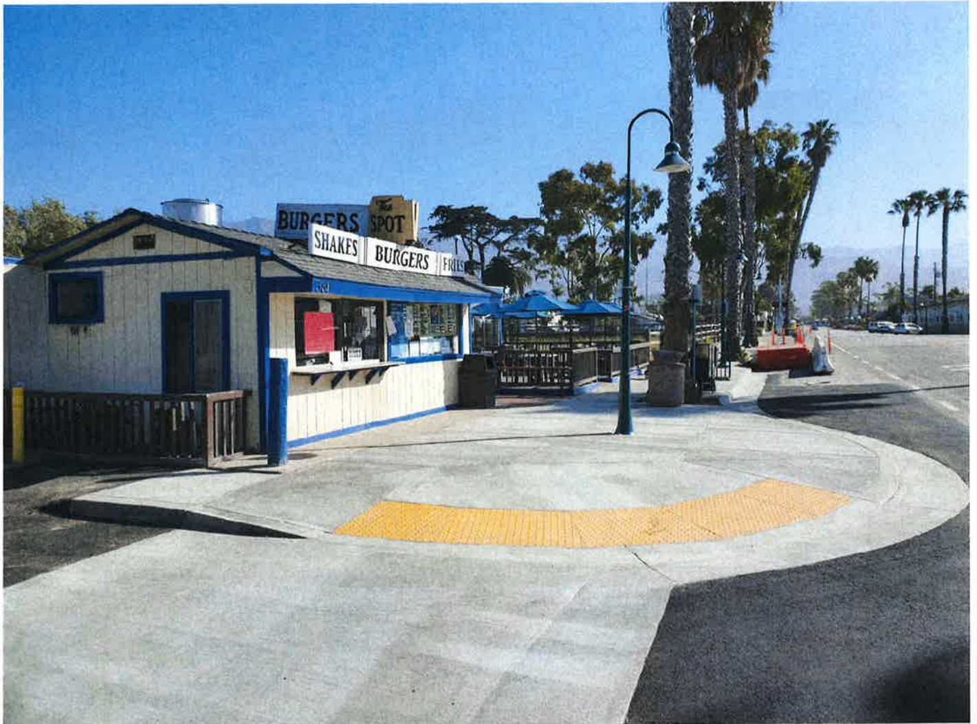
COMPLETED CURB RAMP. NORTH WEST CORNER LINDEN AVE. AND DORRANCE WAY INTERSECTION.
