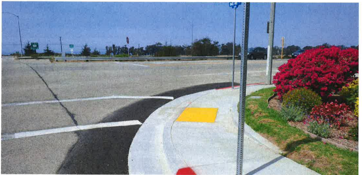
COMPLETED CURB RAMP. NORTH WEST CORNER BAILARD AVE. AND VIA REAL INTERSECTION.
