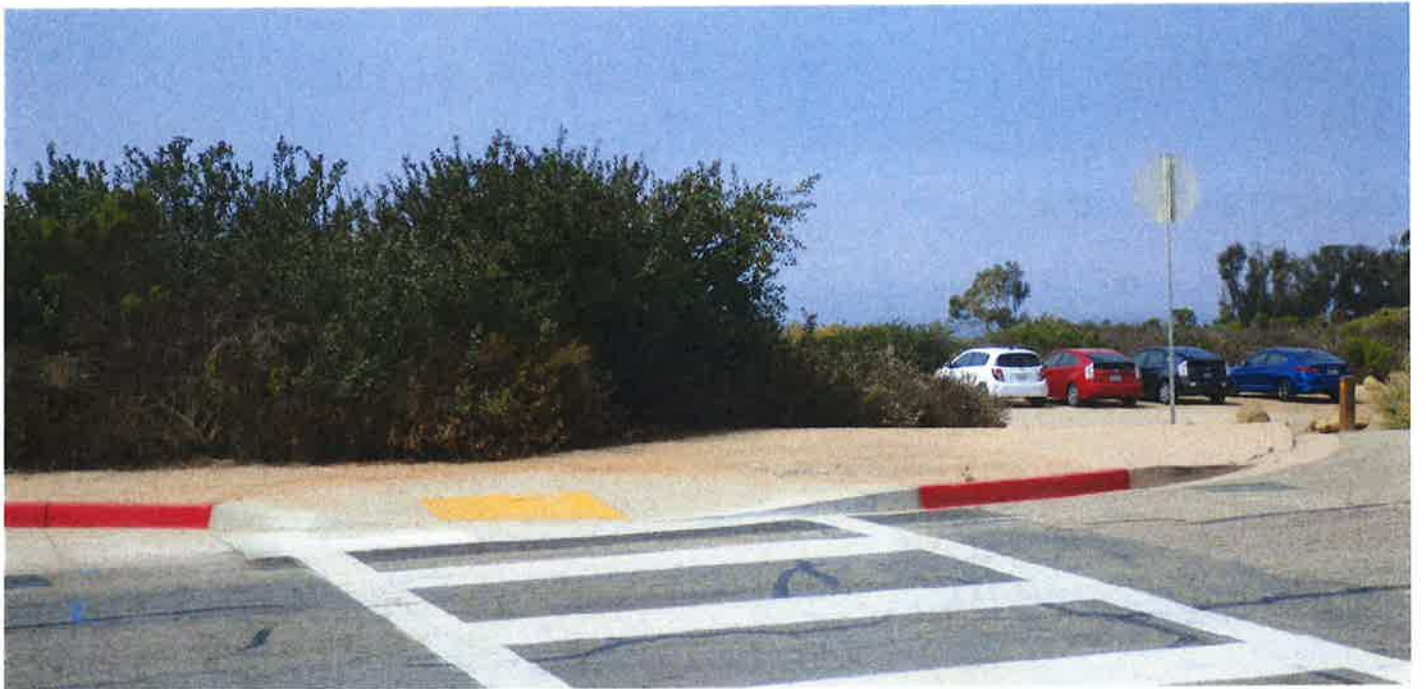
COMPLETED CURB RAMP. SOUTH EAST CORNER BAILARD AVE. AND CARPINTERIA AVE. INTERSECTION.
