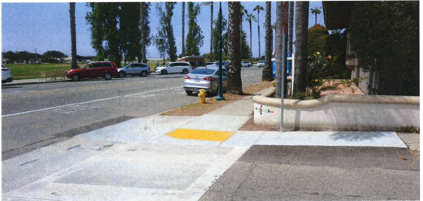
COMPLETED CURB RAMP. SOUTH WEST CORNER LINDEN AVE. AND DORRANCE WAY INTERSECTION.
