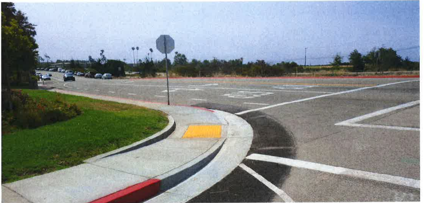
COMPLETED CURB RAMP. NORTH EAST CORNER BAILARD AVE. AND VIA REAL INTERSECTION.
