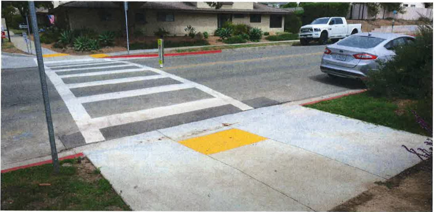
COMPLETED CURB RAMP. NORTH EAST CORNER SANTA YNEZ AVE. AND CATLIN CIR. INTERSECTION.
