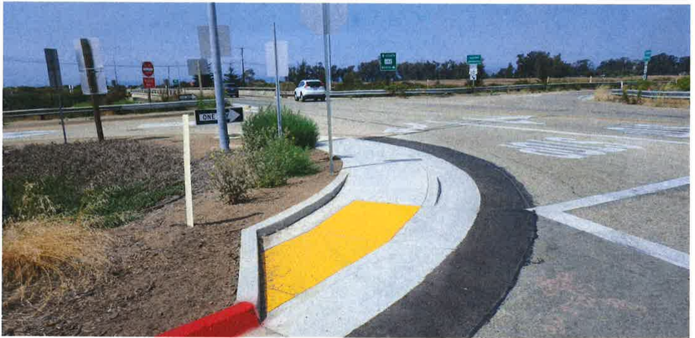
COMPLETED CURB RAMP. SOUTH EAST CORNER BAILARD AVE. AND VIA REAL INTERSECTION.
