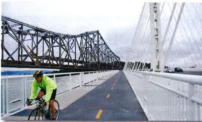
SFOBB SAS Bike Path/Pedestrian Bridge, CA
