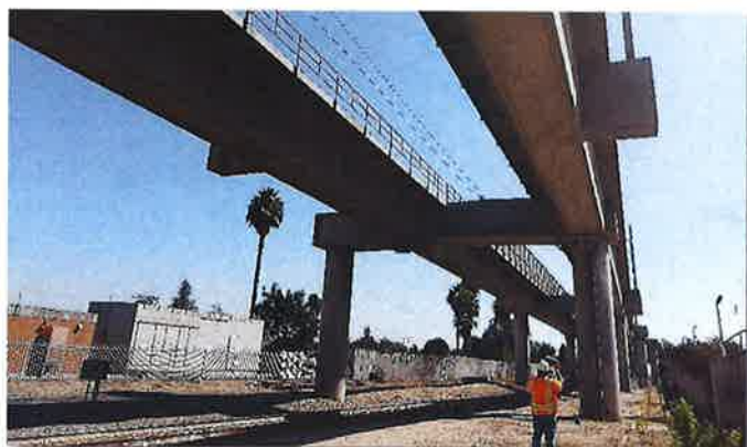
Slauson Bridge in Long Beach, CA, LA Metro. Light Rail Bridge along Blue Line. CIP Concrete Box Girder. Inspection/Repair Recommendations.
