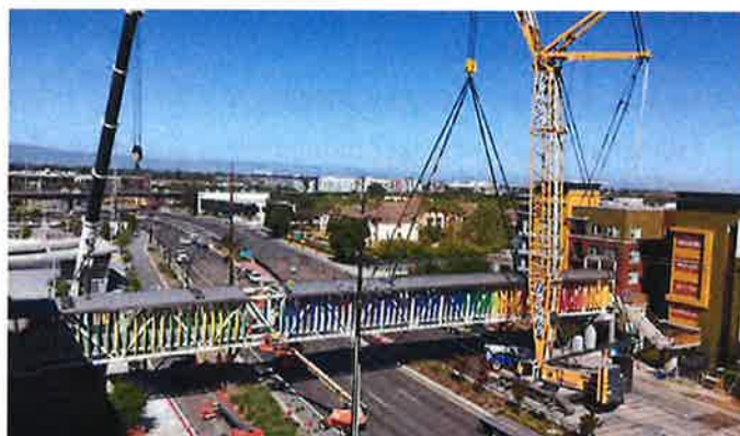
Montague Expressway Pedestrian Overcrossing, Milpitas, CA, VTA. Construction of a New Structural Steel Truss.
