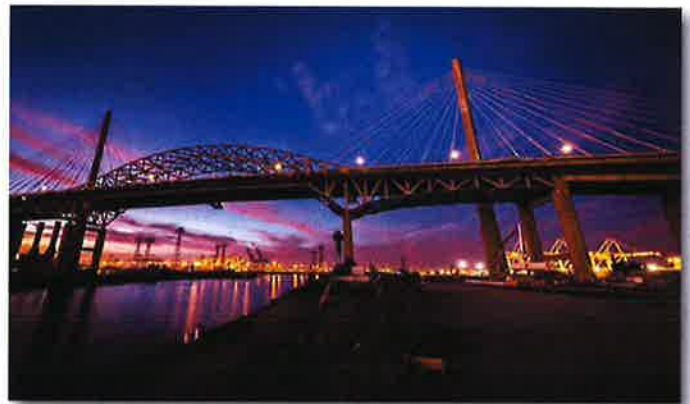
New Gerald Desmond Bridge, Long Beach, CA
