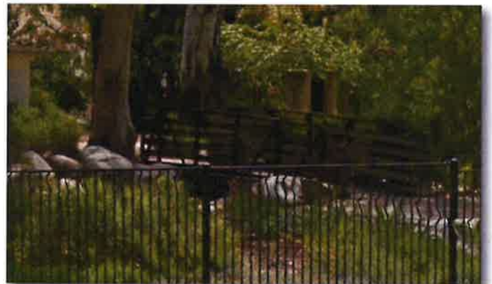
Reyes Adobe Historic Site Pedestrian Bridge, Agoura Hills, CA
