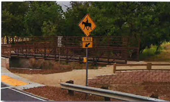
Chesebro Park Bridge (Accessible Pedestrian Bridge), Agoura Hills, CA
