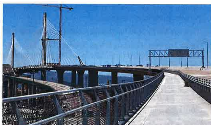
New Gerald Desmond Bridge, Pedestrian Bike Path (GDB), Long Beach, CA
