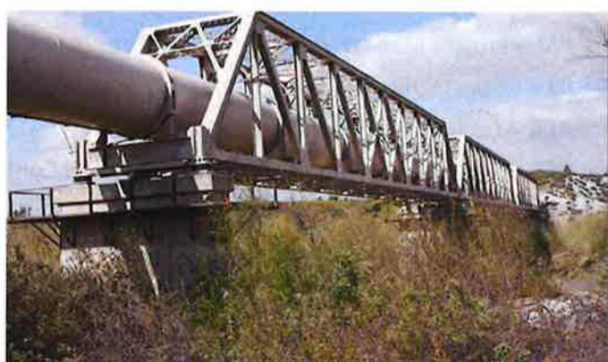
Santa Ana River Crossing in Riverside, CA, MWD. Water Pipe/Maintenance Walkway. Three Structural Steel Trusses. Field Inspection, Seismic Evaluation, and Retrofit.
