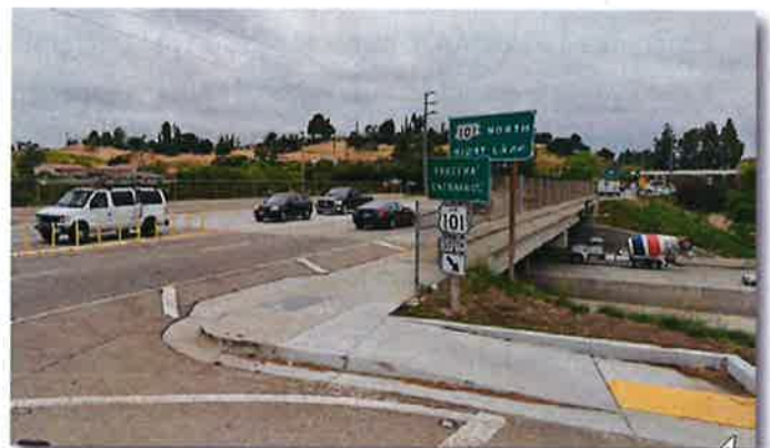
Kanan Road Bridge, Agoura Hills, CA
