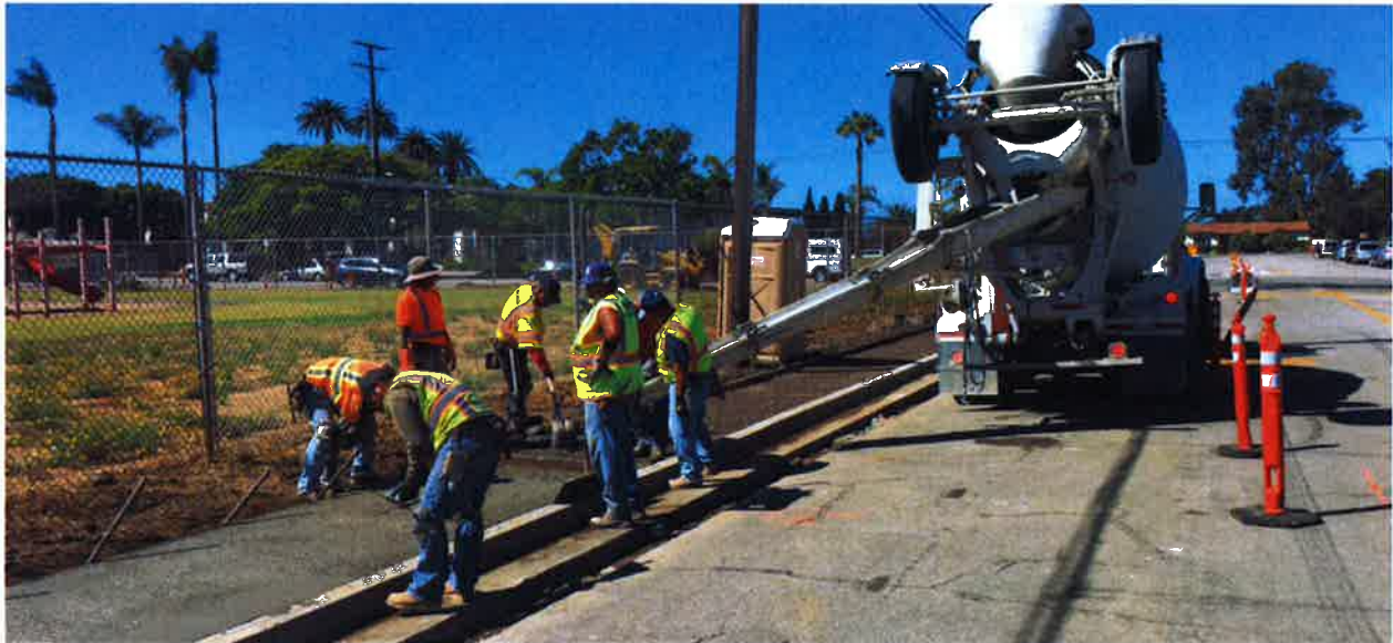
Figure 2 Construction of new sidewalk along Walnut Ave.
