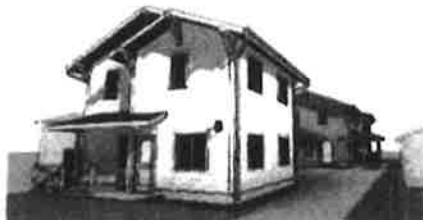
Habitat for Humanity Residences
