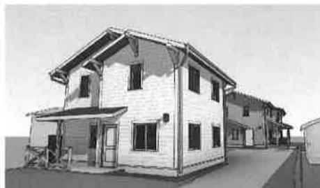
Habitat for Humanity Residences
