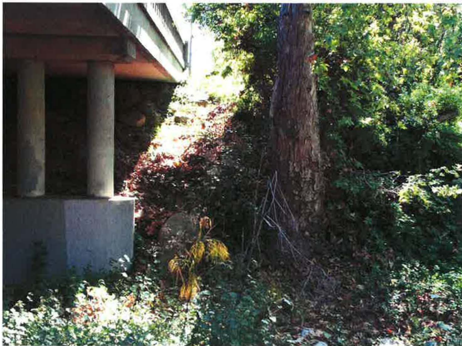
Carpinteria Creek South Bridge East Span
