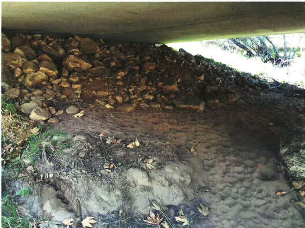
Figure 4: Existing RSP on East Bank of Carpinteria Creek at US 101
