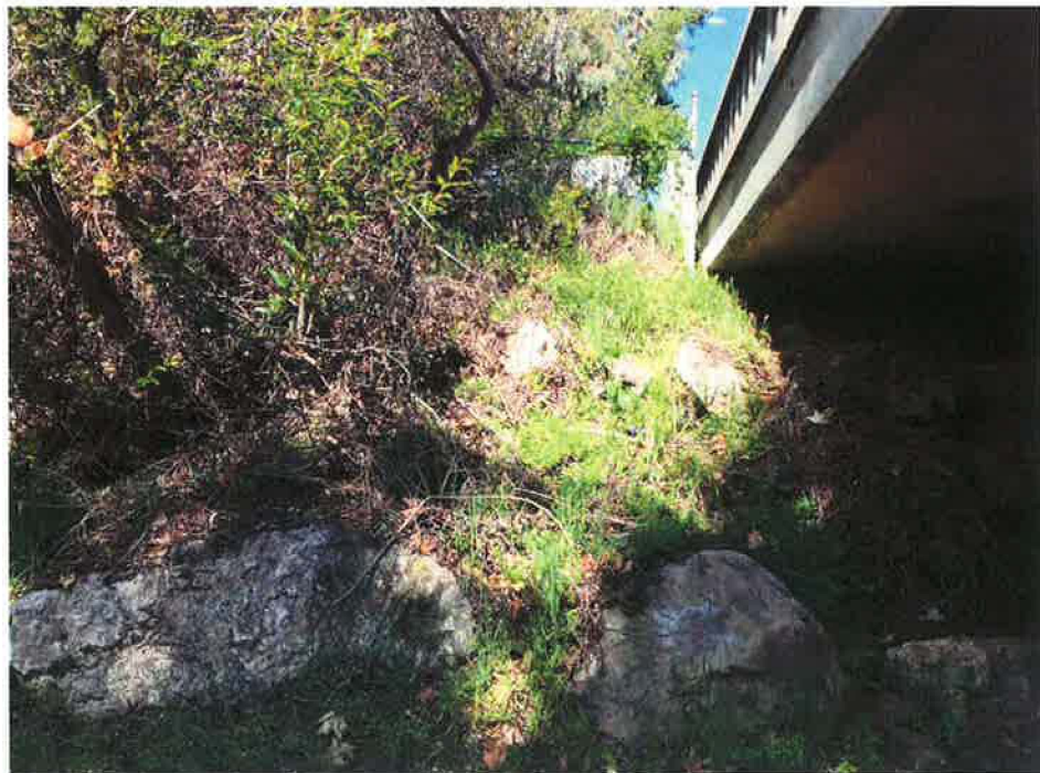
Carpinteria Creek South Bridge West Span
