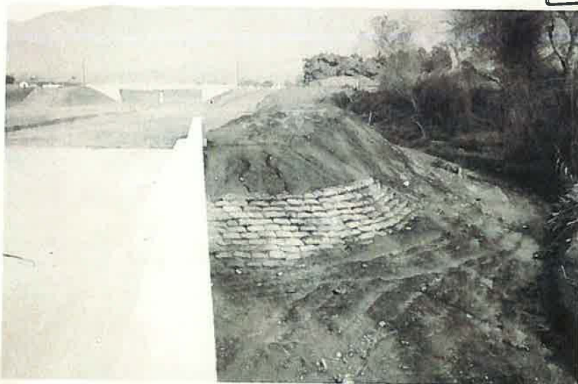
BRS 143-7 Along US face toward EWO dike on RB to prevent over- flow thru thoro cut to Franklin Cr
