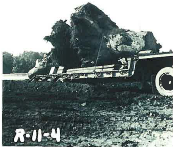
Drift removed from Channel
