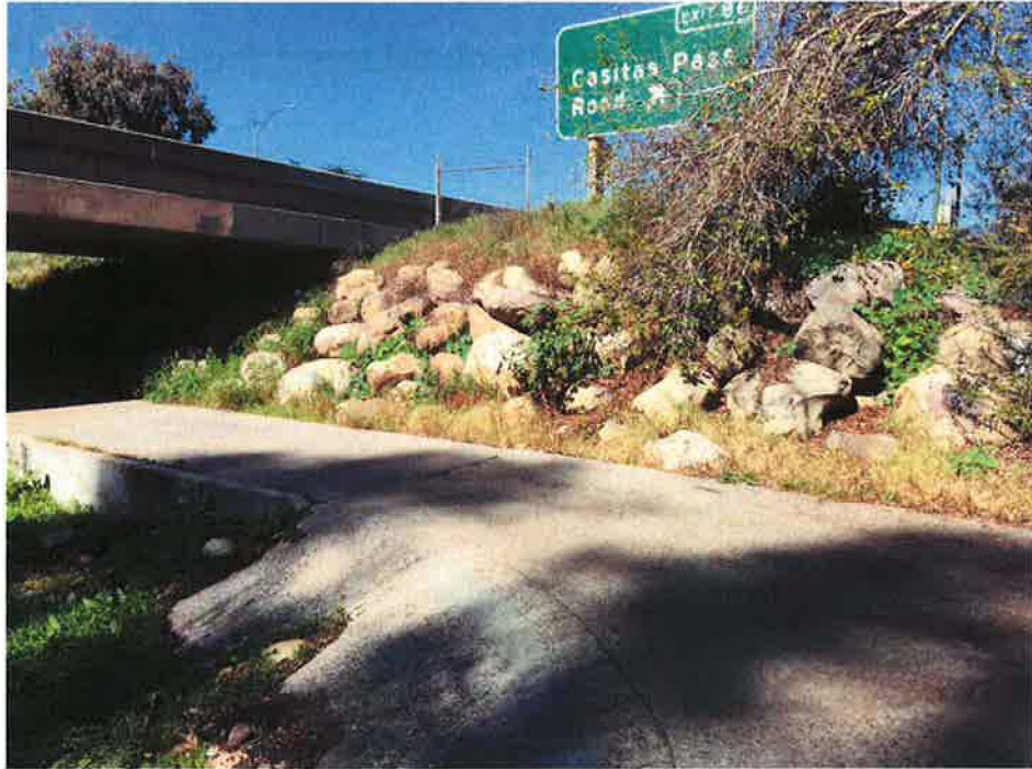
Carpinteria Creek North Bridge West Span
