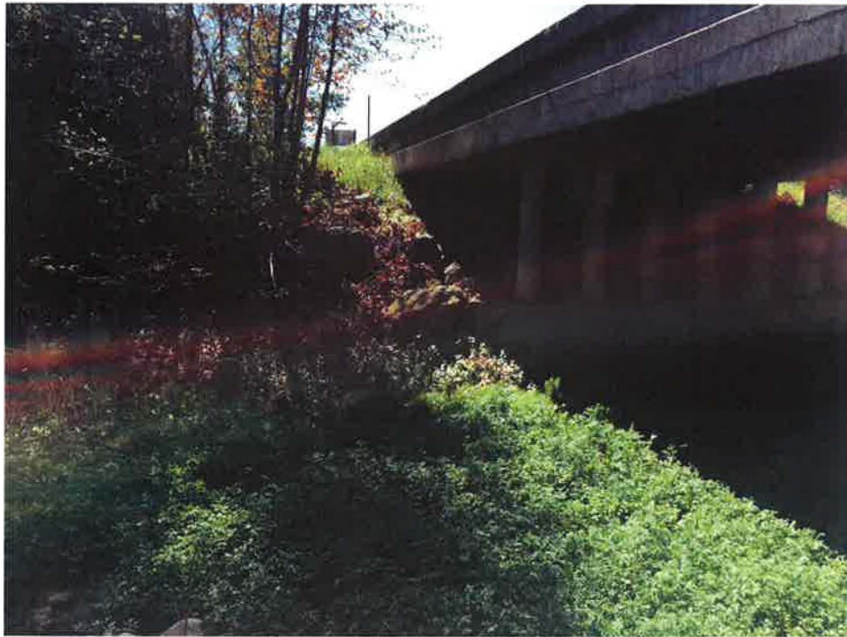
Carpinteria Creek North Bridge East Span
