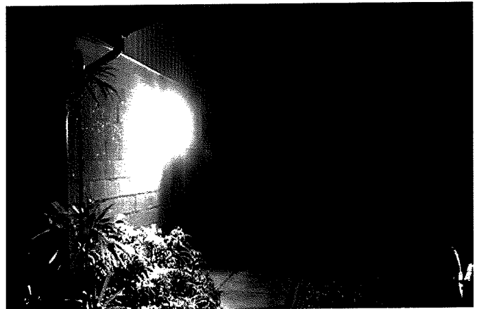
Figure 22: Light fixture that is not shielded creates safety issues (Image Source: International Dark Sky Association)
