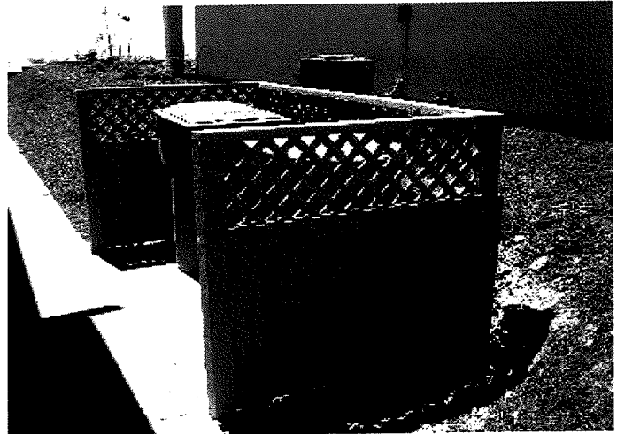
Figure 26: Trash enclosure for solid waste containers
