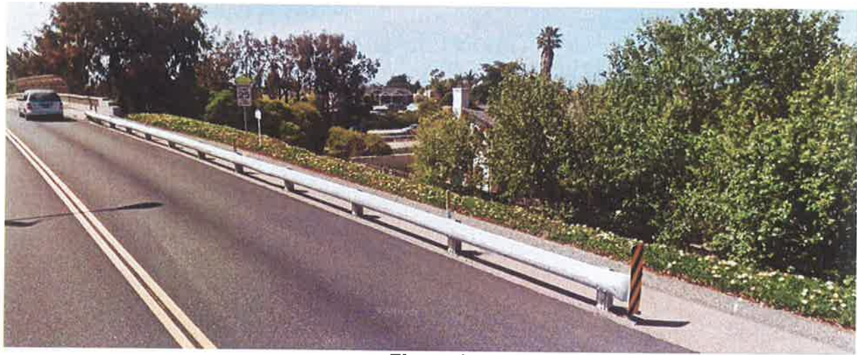
Figure 1. Original Santa Ynez "Half-Moon" Style Guardrail
