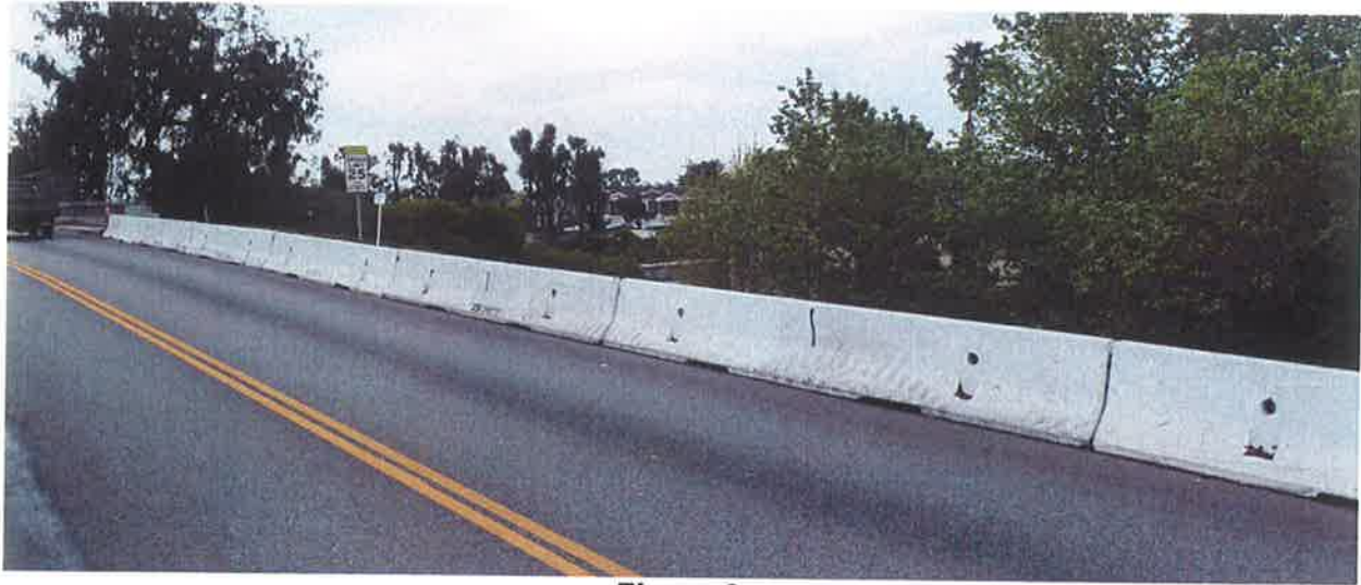
Figure 3. Santa Ynez Guardrail Temporary K-Rail Repair
