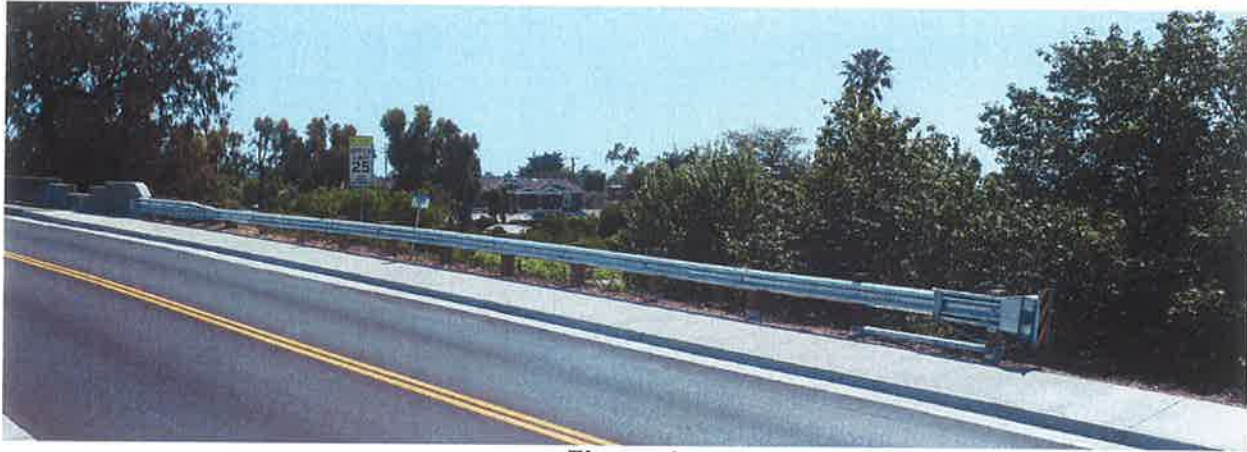
Figure 4. Santa Ynez Guardrail Completed
