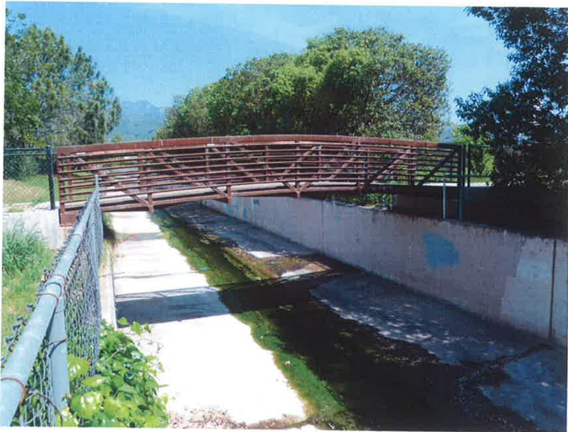
Figure 1 Mission Terrace Pedestrian Bridge over Franklin Channel
