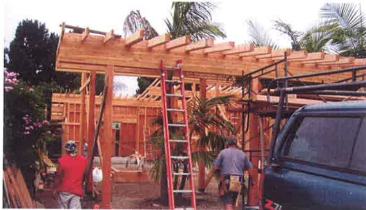
Damiani Residence under Construction
