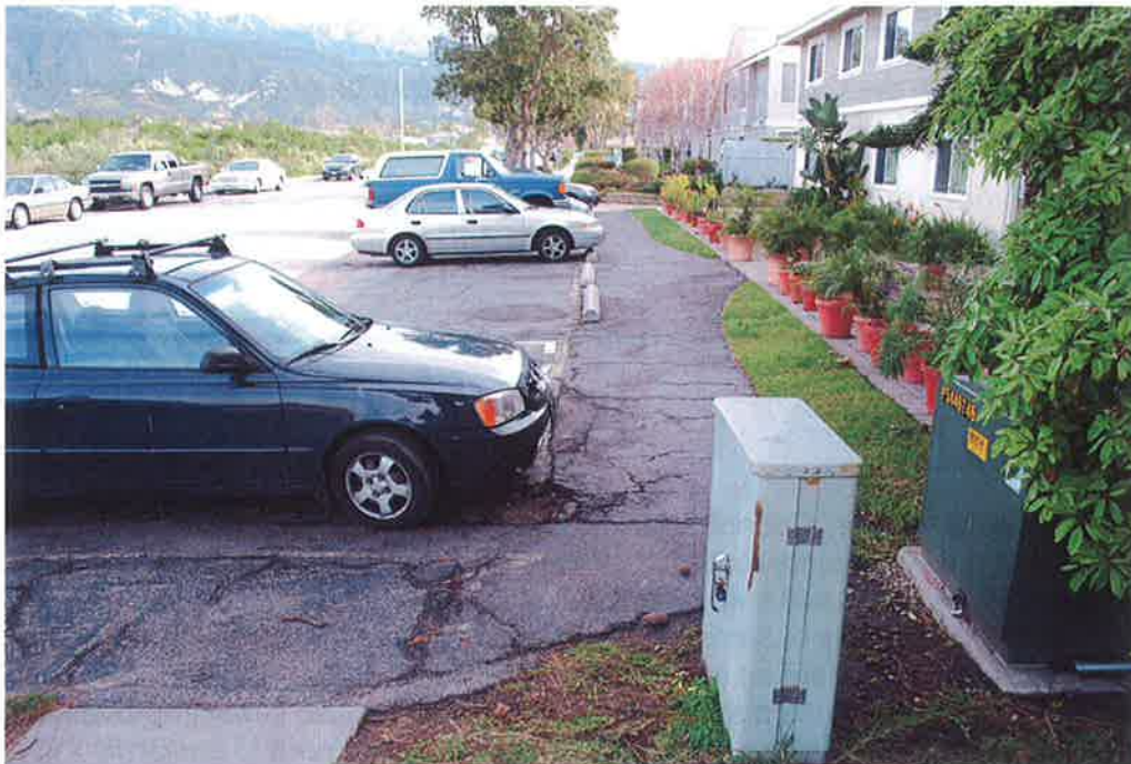
Figure 1 – Sidewalk In-fill location on east side of Ash Avenue between Sandyland Road and 3 rd Street
