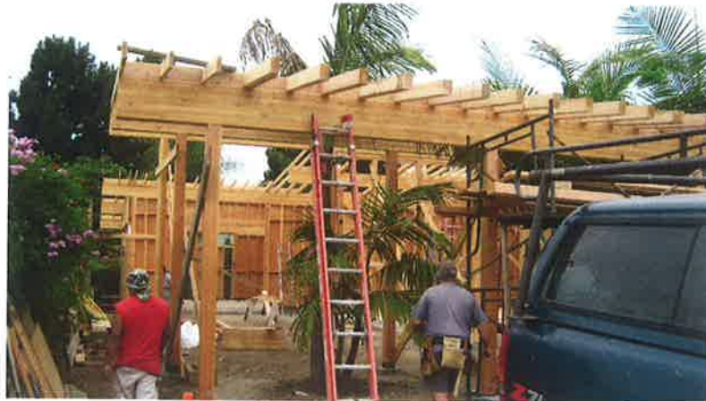
Damiani Residence under Construction
