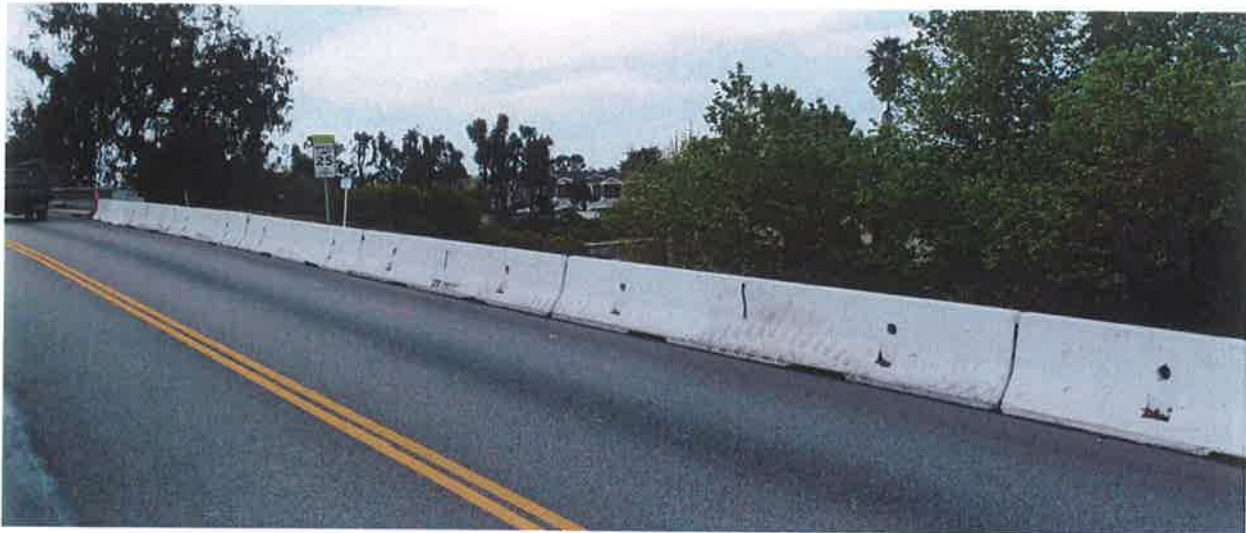
Figure 3. Santa Ynez Guardrail Temporary K-Rail Repair
