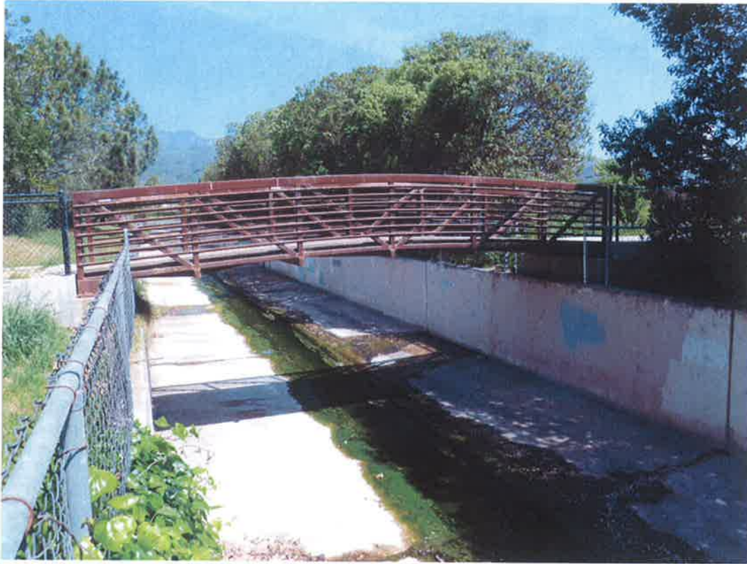
Figure 1 Mission Terrace Pedestrian Bridge over Franklin Channel
