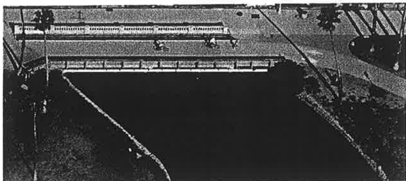
Aerial View of the "Beach way" portion of the Cabrillo Blvd Bridge, Santa Barbara, CA
