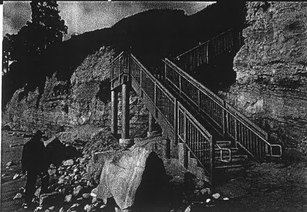
Md Wahiduzzaman inspects completed structure.
