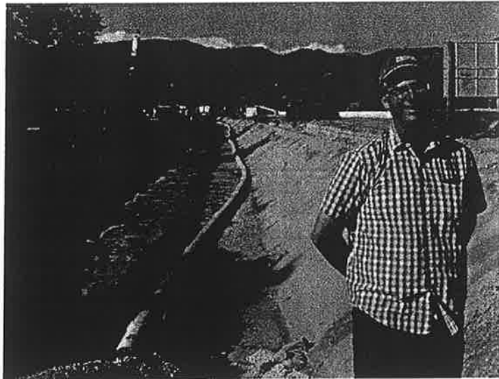
Mr. Onishuk recently led the design of the $20 million San Jose Creek Capacity Improvement and Fish Passage Project currently under construction in Goleta.
