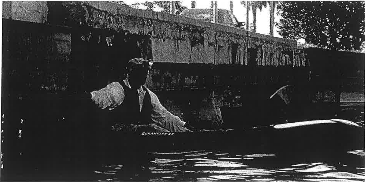
Md. Wahiduzzaman inspects Cabrillo Blvd. Bridge.
