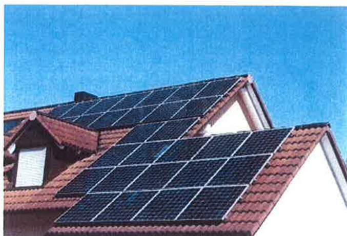
Figure 31: Example of a residential photovoltaic system.
