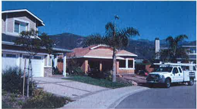
The residence on Lot 18 under construction
