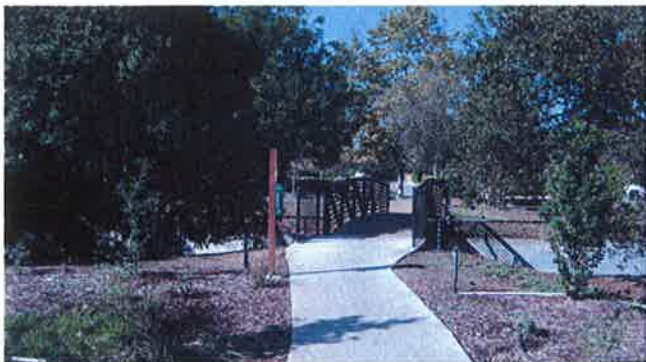
Looking over the footbridge to Franklin Creek Park
