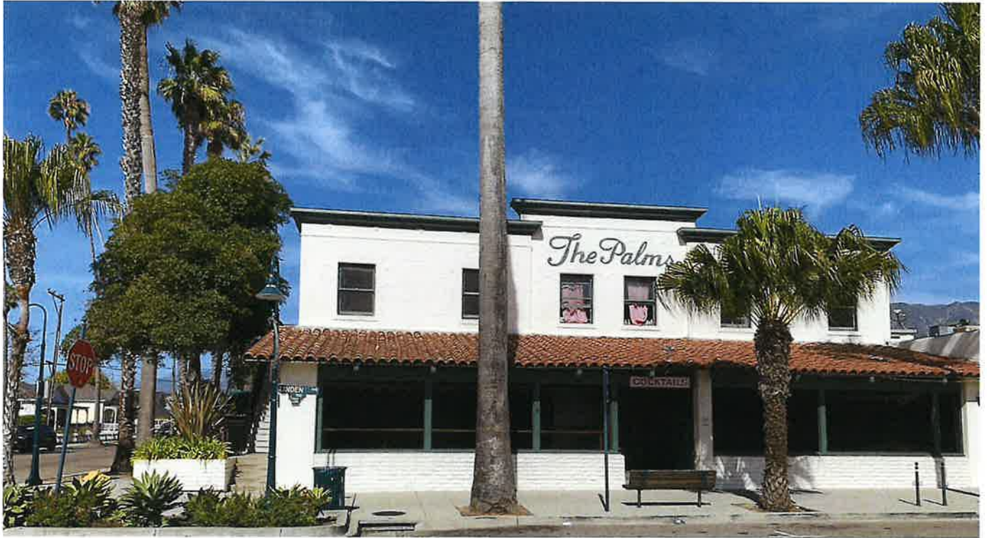
Exhibit 1, Existing Signage on the Street Façade facing Linden Avenue (installed in the early 1960s)
