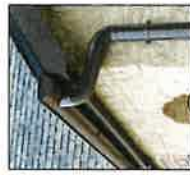
3" HALF-ROUND GUTTER, 3" DOWNSPOUT
