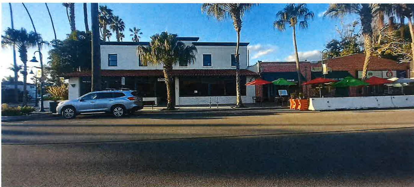
Exhibit 6, The east elevation facing Linden Avenue, looking west (November 2023)
