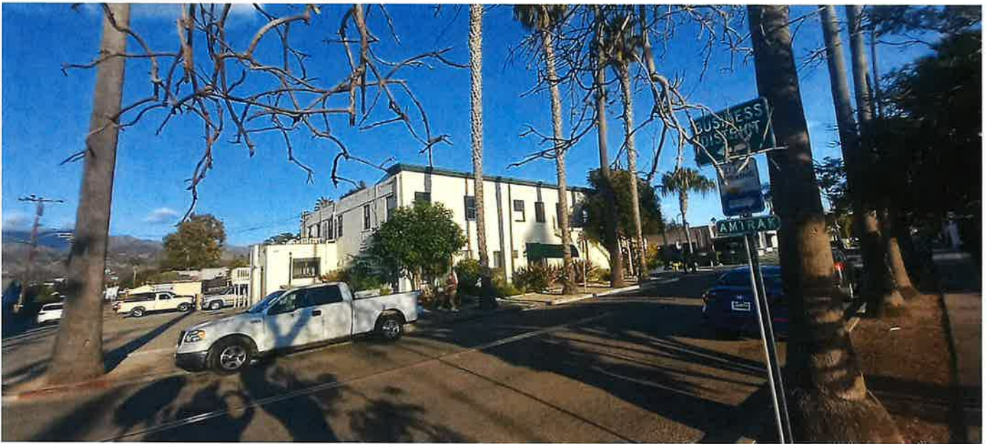
Exhibit 16, South and west elevations. looking northeast (November 2023)
