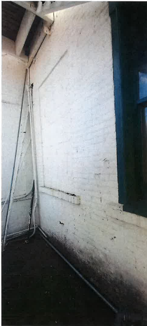
Exhibit 25, Infilled window opening on the north elevation of the one-story portion of the elevation, looking southeast, (November 2023)
