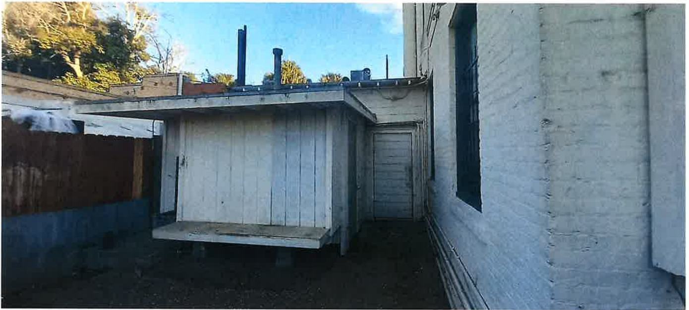
Exhibit 23, North end of the west elevation, with a detail of the non-contributing wood frame additions to the west end of the one-story wing (November 2023)
