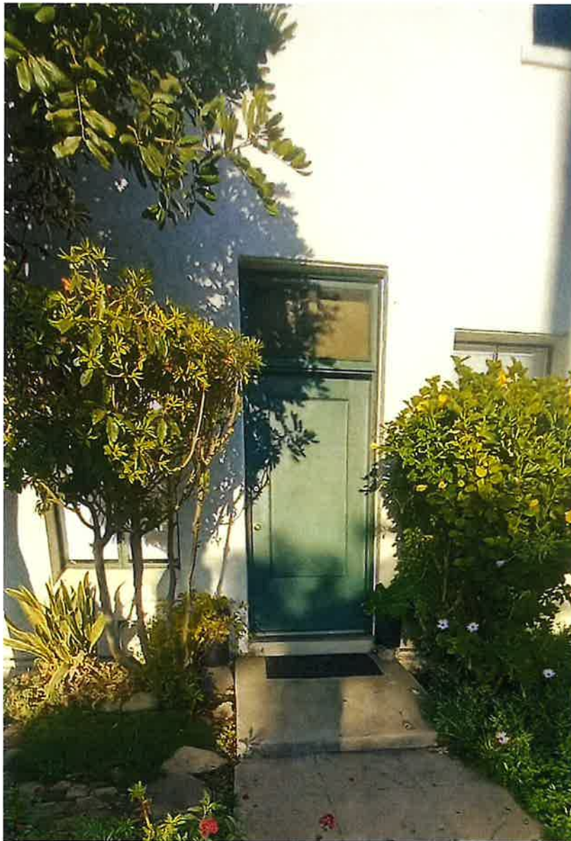
Exhibit 14, South elevation, with a detail of the door at the west end of the elevation, looking north (November 2023)
