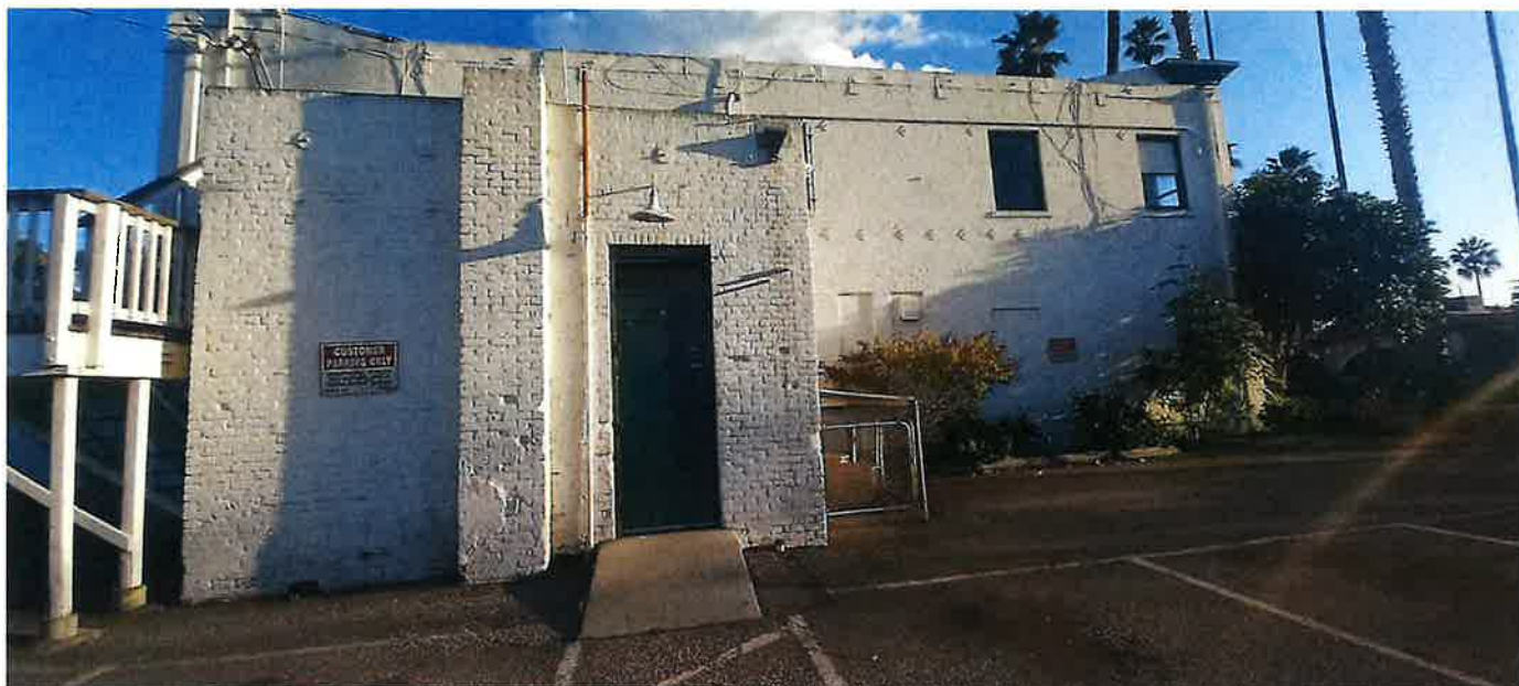
Exhibit 20, North end of the west elevation, looking east (November 2023)
