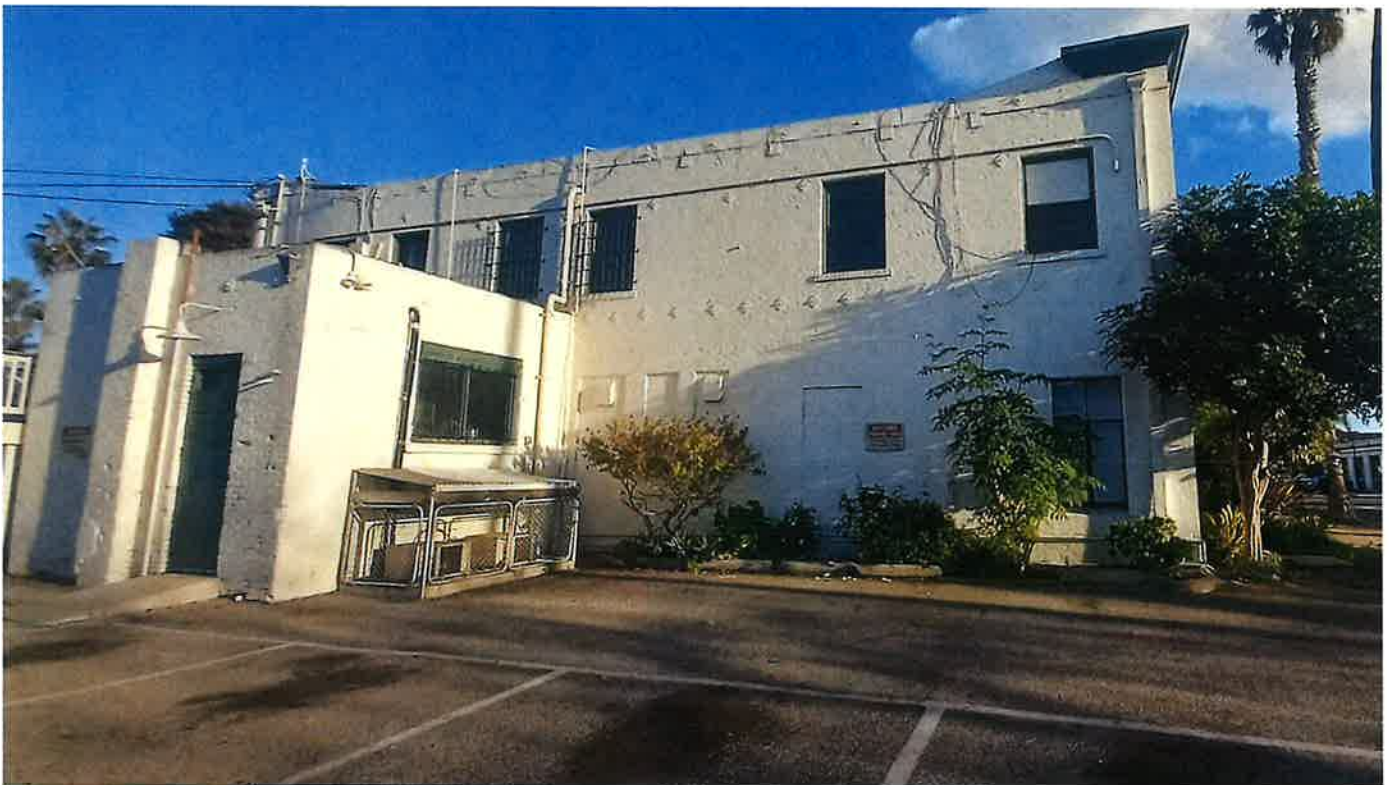
Exhibit 19, South end of the west elevation, looking east (November 2023)
