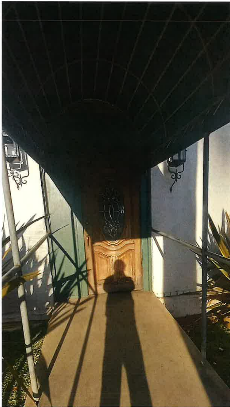
Exhibit 15, South elevation, with a detail of the non-original door and canopy near the center of the elevation, looking north (November 2023)
