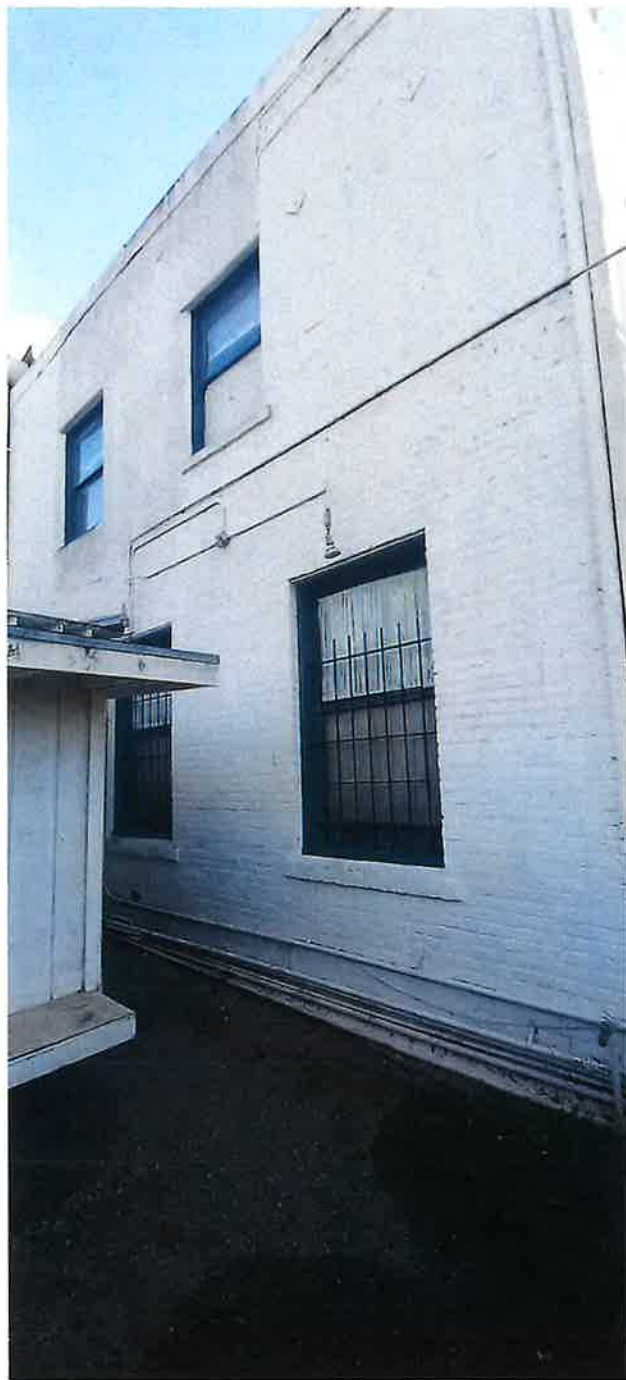
Exhibit 26, West end of the north elevation, looking southeast, (November 2023)
