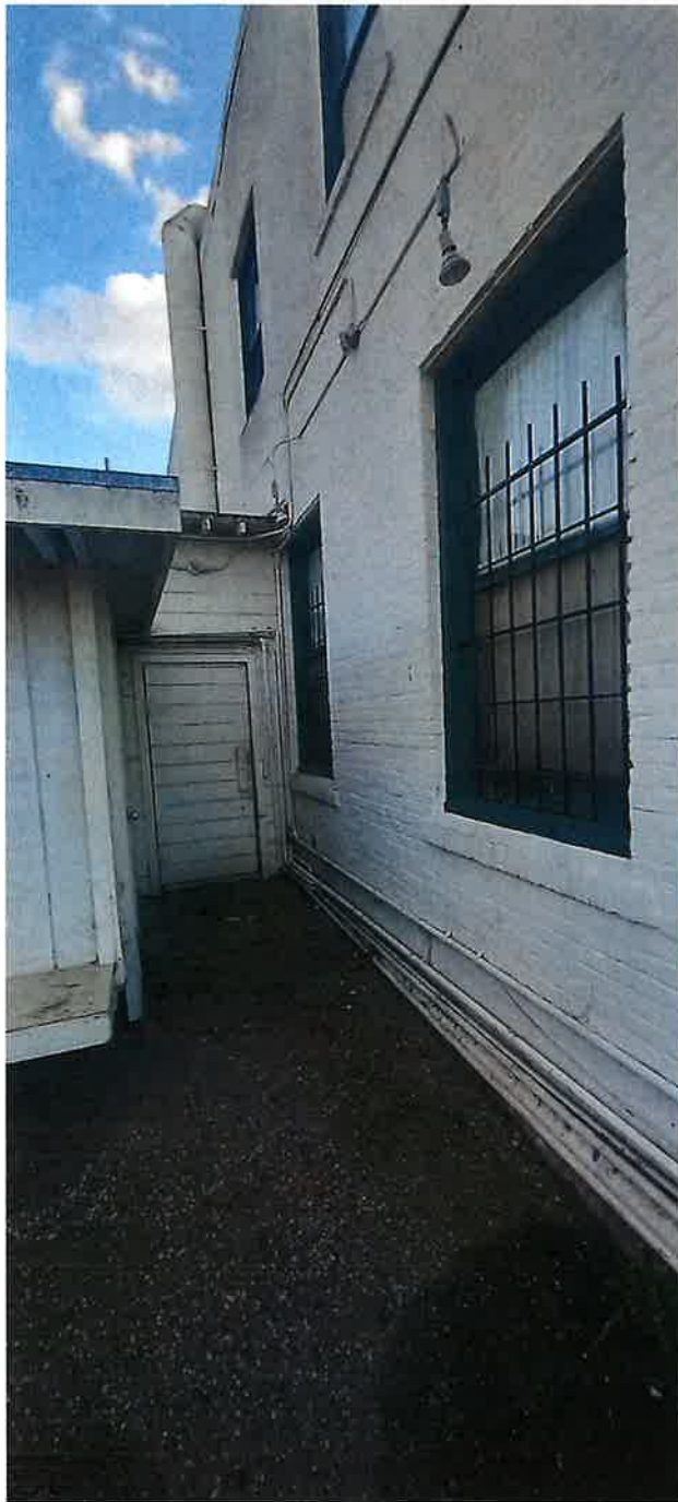
Exhibit 27, West end of the north elevation, looking southeast, (November 2023)
