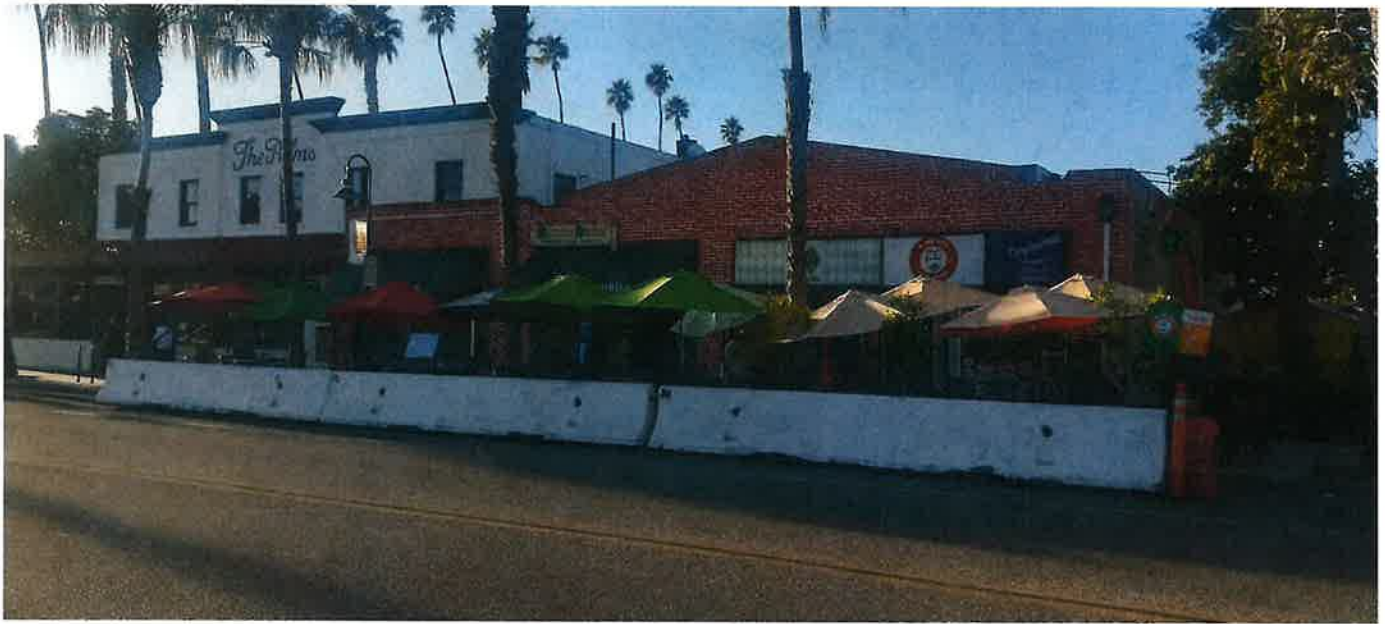
Exhibit 3, The west side of the 700 Block of Linden Avenue with the Palms to the left, looking southwest (November 2023)
