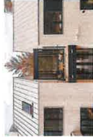
METAL RAILING/GUARDRAIL WITH W/TE MESH INFILL 1 1/2" O.D. 1.5" SCH. 40 STEEL PIPE AS ASTER GUARD RAIL/FALLING WITH W/TE MESH INFILL FINISH: BLACK
