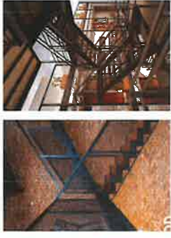
METAL RAILING/GUARDRAIL WITH W/TE MESH INFILL 1 1/2" O.D. 1.5" SCH. 40 STEEL PIPE AS ASTER GUARD RAIL/FALLING WITH W/TE MESH INFILL FINISH: BLACK
