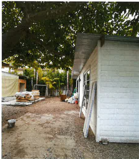
⑫ LOOKING AT NORTH ELEVATION FROM PROJECT SITE
