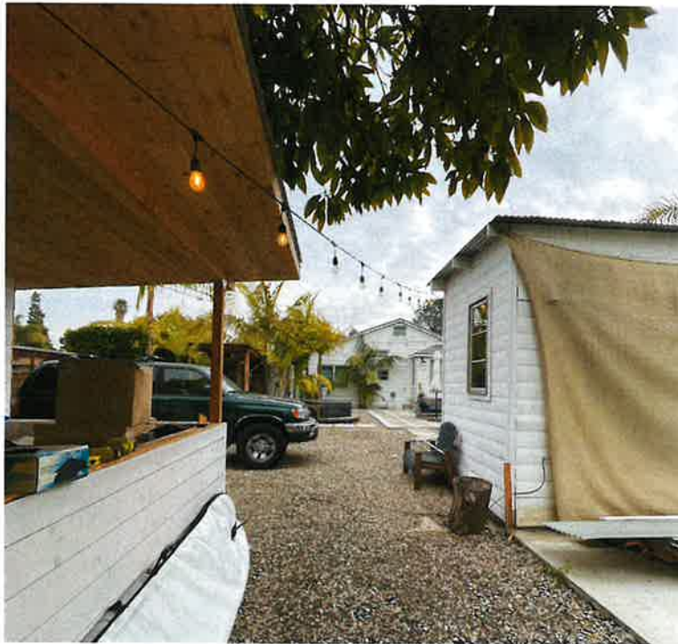
③ LOOKING AT WEST ELEVATION FROM PROJECT SITE
