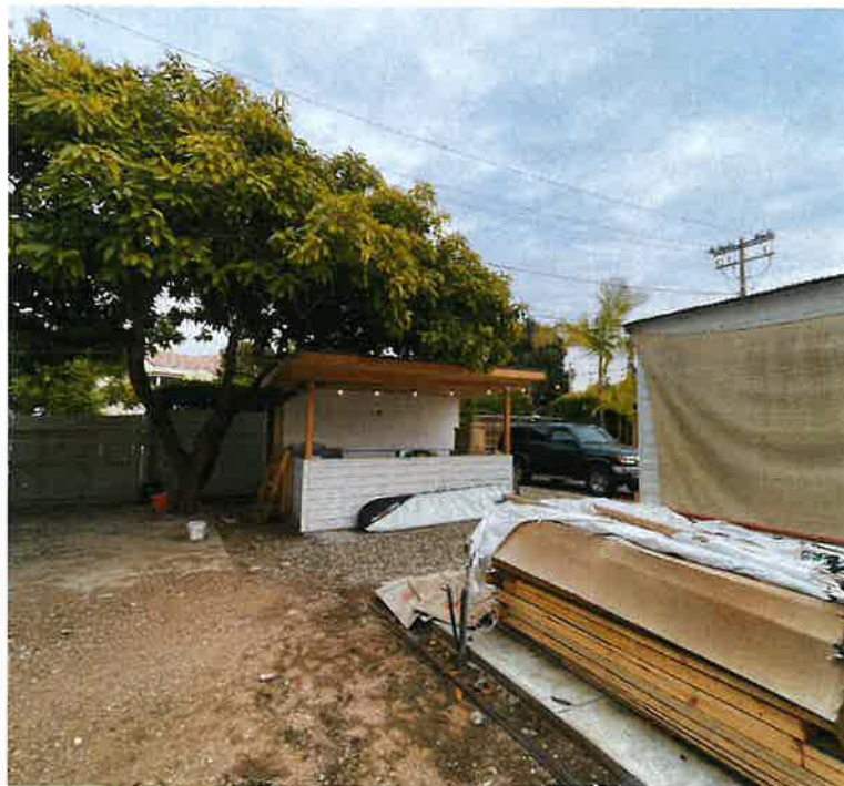
② LOOKING AT SOUTH ELEVATION APPROACHING (E) WET BAR FROM PROJECT SITE
