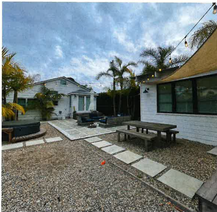
④ APPROACHING WEST ELEVATION OF MAIN RESIDENCE FROM PROJECT SITE
