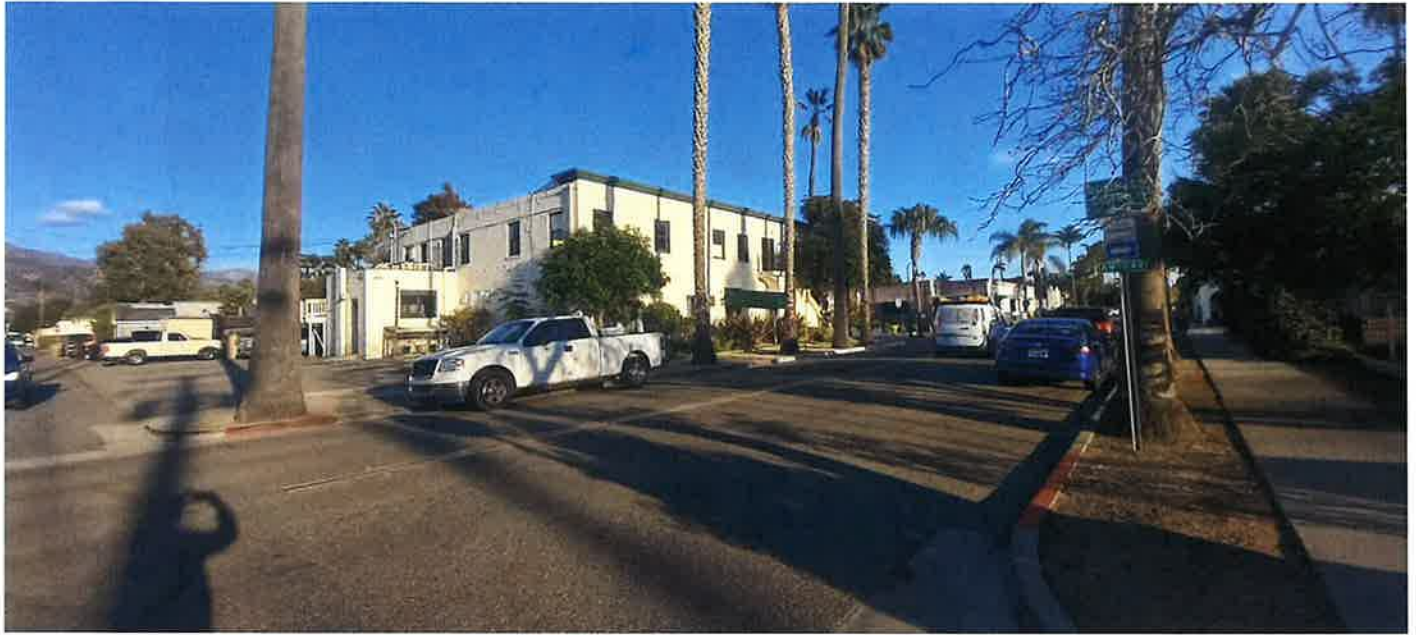
Exhibit 11, South and west elevations, with 7 th Street in the foreground (November 2023)
