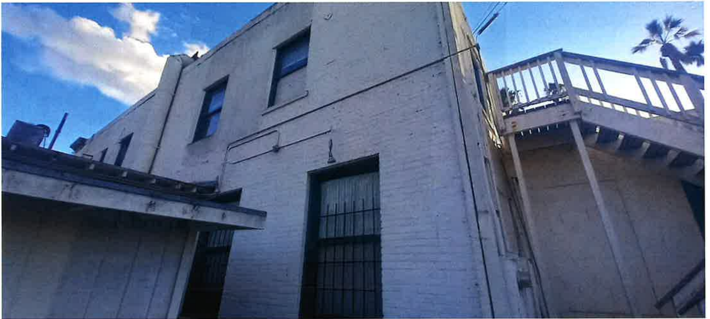
Exhibit 28, West end of the north elevation, looking southeast, (November 2023)
