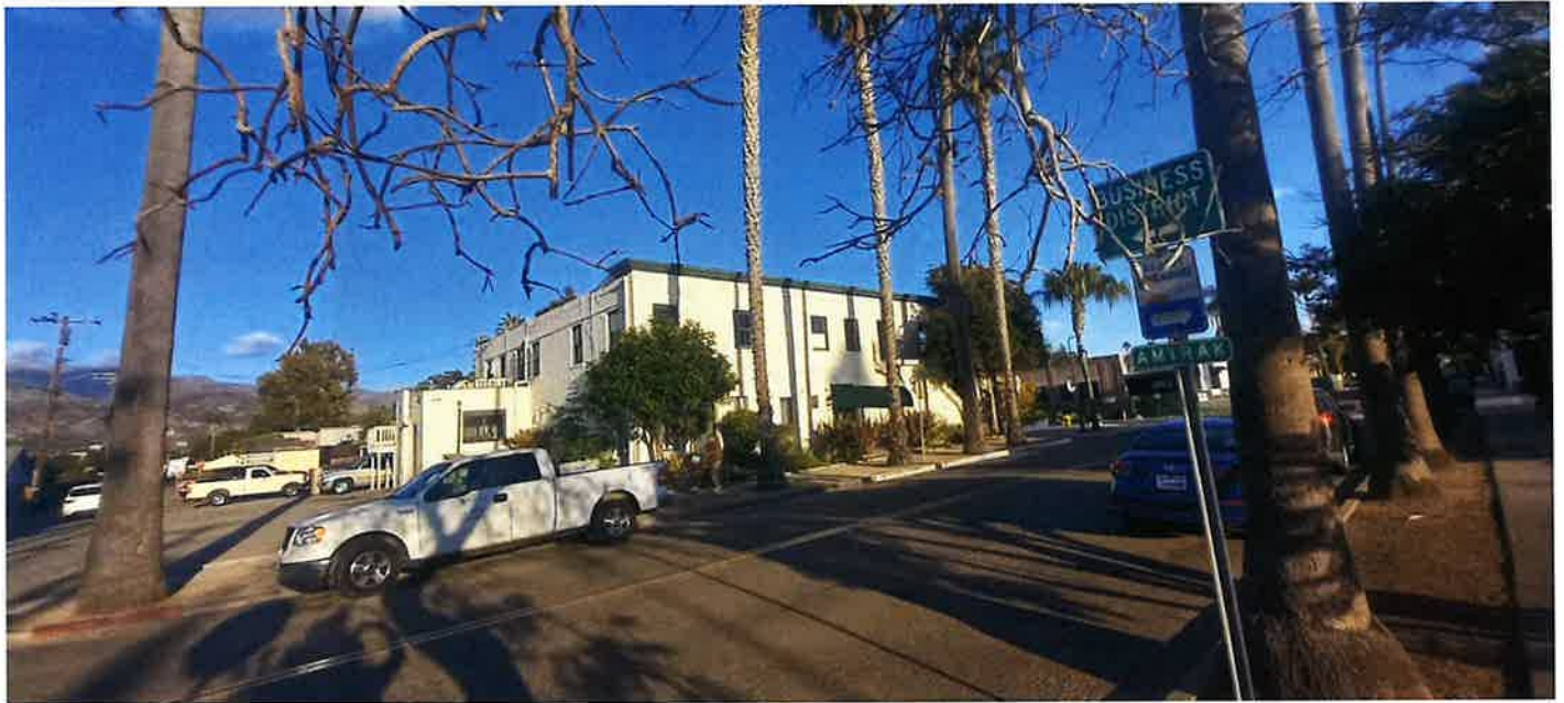
Exhibit 16, South and west elevations. looking northeast (November 2023)
