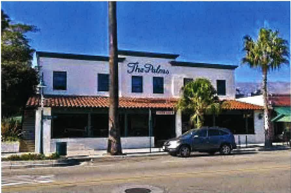
Figure 6, The Palms After the 1987 Renovations (Photo: Circa-2000)
