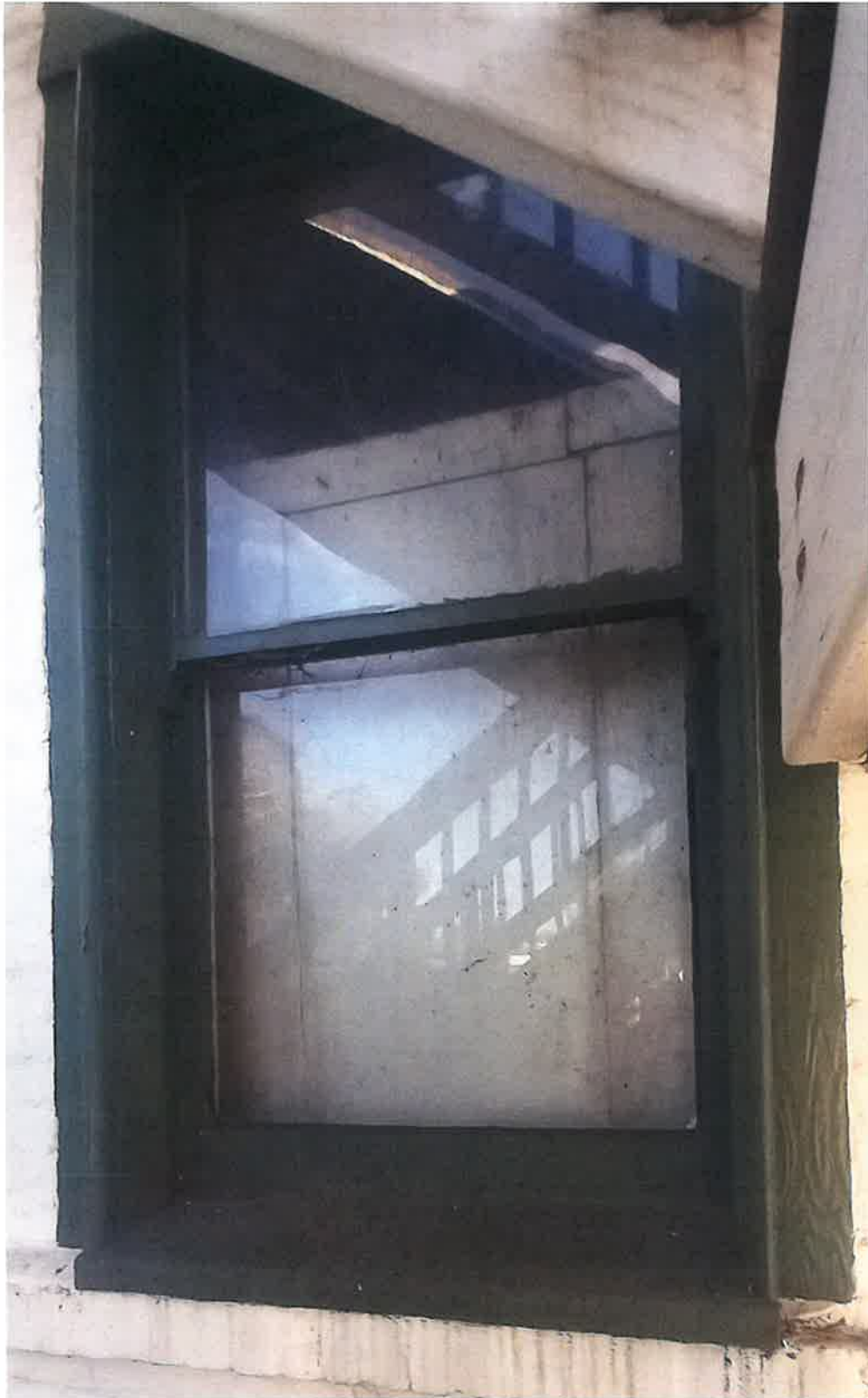
Exhibit 6a, Example of the building's original wood double hung wood sash unit (November 2023)
