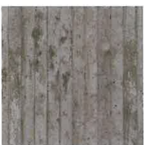
CN-1 BOARD-FORMED CONCRETE
