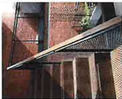
12 GUARDRAIL 1 1/2" O.D. 1.5" SCH. 40 STEEL PIPE AS ASTM GUARD RAIL/RAILING WITH WIRE MESH INFILL FINISH: BLACK
