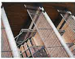
12 GUARDRAIL 1 1/2" O.D. 1.5" SCH. 40 STEEL PIPE AS ASTM GUARD RAIL/RAILING WITH WIRE MESH INFILL FINISH: BLACK
