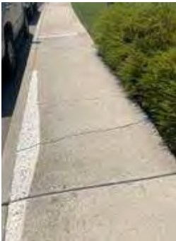
Hazard 4: 5372 Santa Rosa Ln
