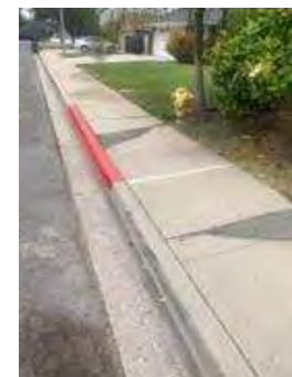
Hazard 18: 5420 Granada Way
