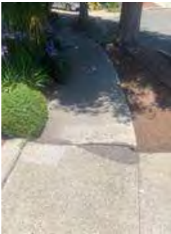
Hazard 3: 1547 Myra St
