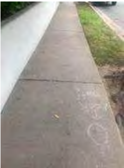
Hazard 9: 1493 Trenora St
