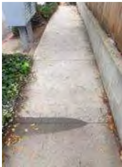
Hazard 13: 1306 La Manida St
