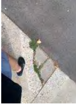
Hazard 9: 1536 Linden Ave
