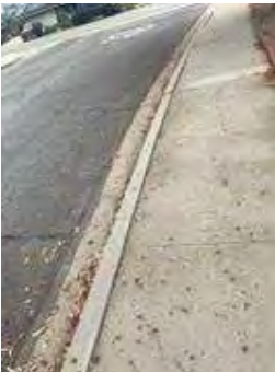
Hazard 20: 5404 Granada Way C^sw
