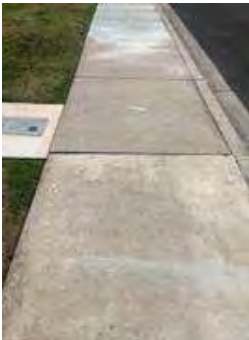
Hazard 1: 5371 Santa Rosa Ln
