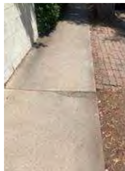
Hazard 8: 1477 Noma St
