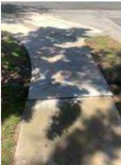
Hazard 1: 5444 Dariesa St
