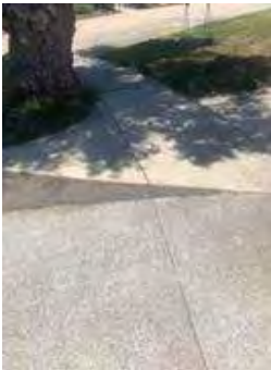
Hazard 1: 1546 Myra St
