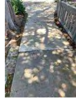
Hazard 12: 5378 Dariesa St
