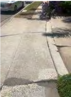
Hazard 4: 1547 Myra St
