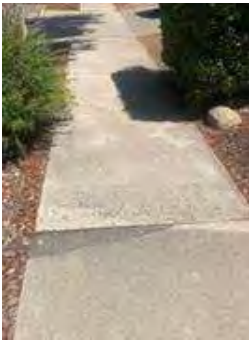
Hazard 19: 5451 Shemara St
