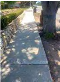
Hazard 4: 5458 Dariesa St
