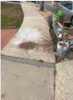
Hazard 1: 1477 Andrea St
