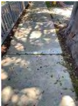
Hazard 13: 5378 Dariesa St
