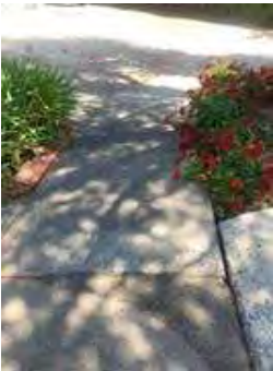
Hazard 3: 1488 Alva St
