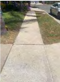
Hazard 5: 5458 Dariesa St
