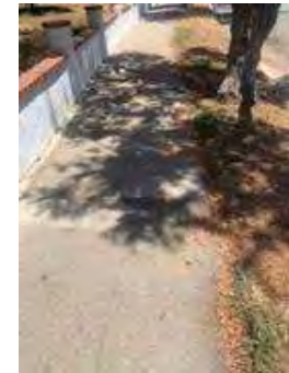
Hazard 6: 1478 Noma St
